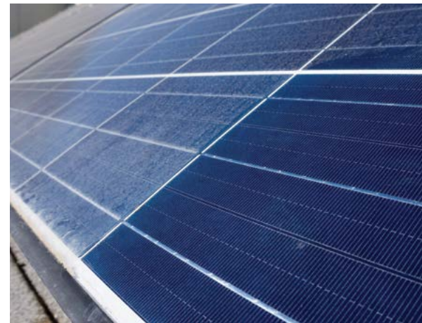
Figure 7. Uniform soiling pattern commonly found on large systems.
